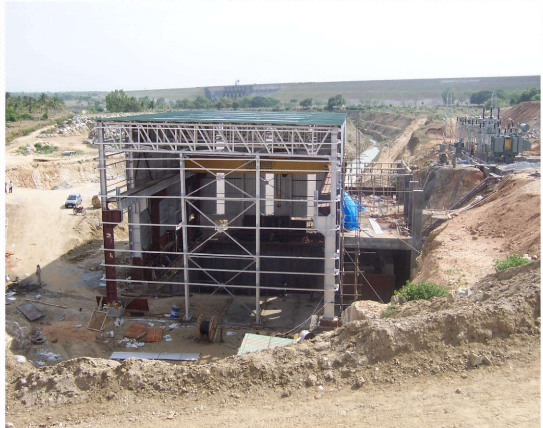
POWER HOUSE, HEMAVATHI POWER PLANT
