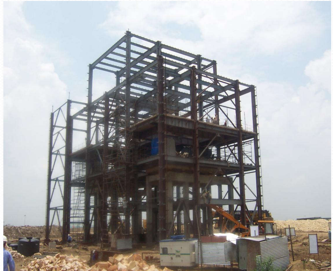
CRUSHER HOUSE, EMCO POWER PLANT
