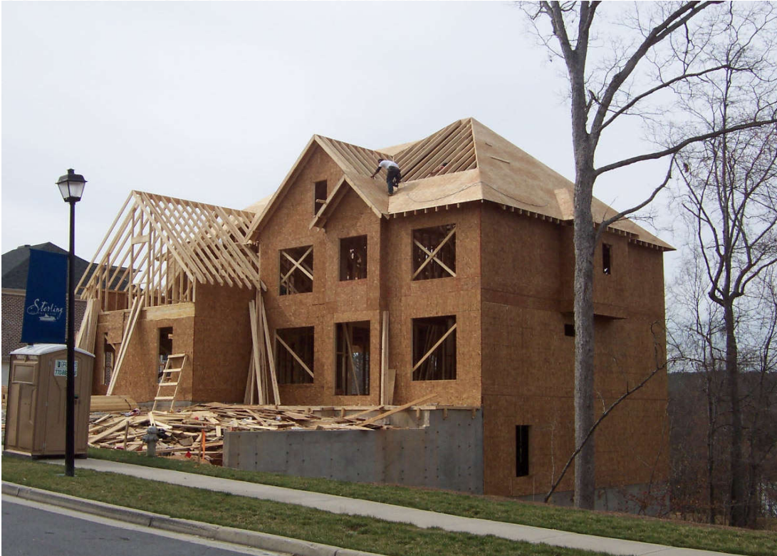
RESIDENTIAL BUILDING UNDER CONSTRUCTION, NASHVILLE
