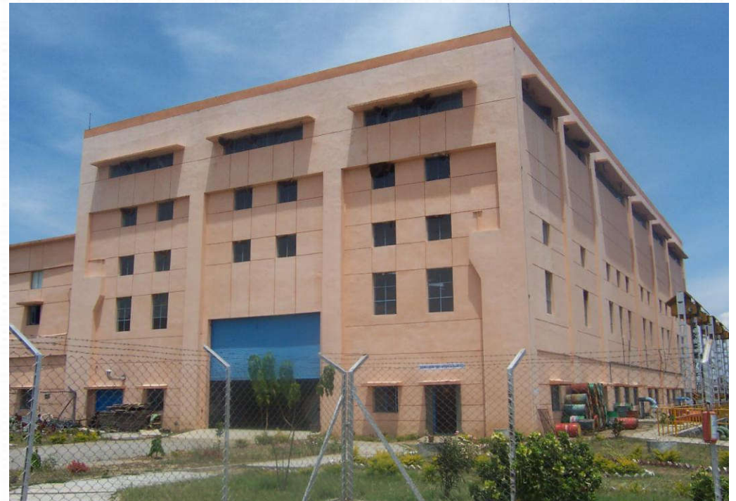
2x9 MW KABINI HYDRO POWER PLANT, POWER HOUSE
