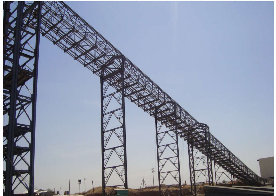
CONVEYOR GALLERY & TRESTLE FOR INDIA BULLS
